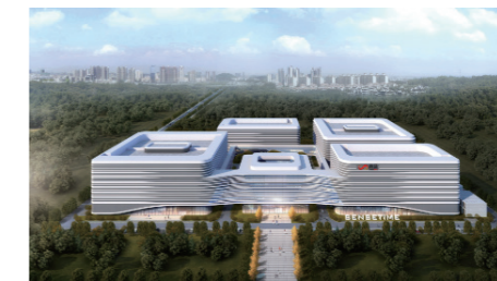
External Design of SenseTime AIDC
